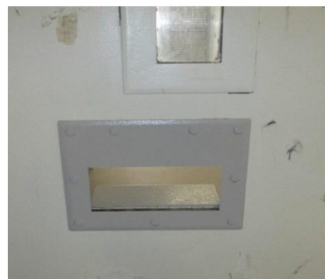
Image 28: View of a cuff trap from inside a young person’s room. People using this communication may bring a chair to the door, so they are at face level with the cuff trap.
